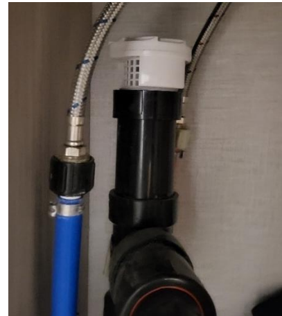
Figure 154. Air admittance valve.
