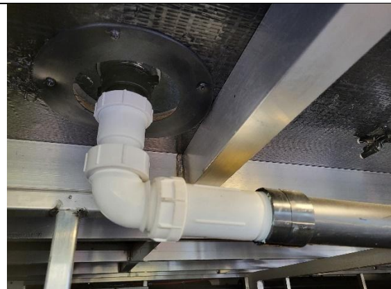
Figure 153. Waterless p-trap under a shower location.
